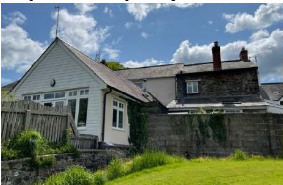
Image of rear wing facing south-east
