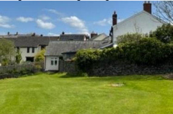
Image of rear wing facing east
