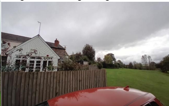
Image of rear wing facing south-west
